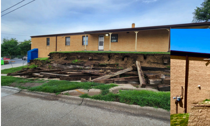
Retaining Wall on Calhoun Street
